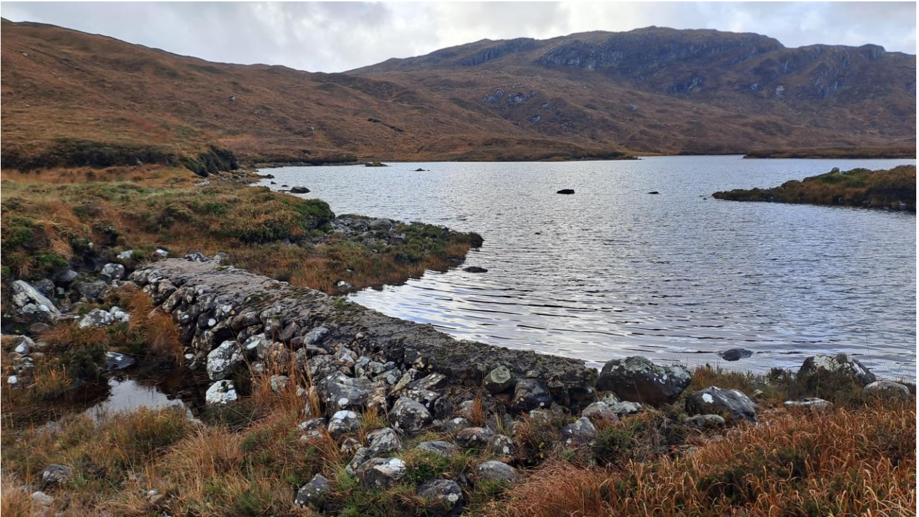
Plate 8 – SLR101, the northern portion of the weir
