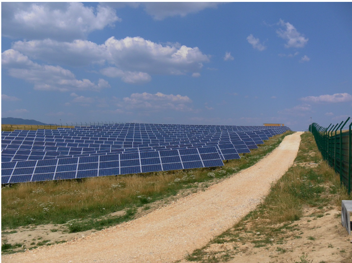
Solpark i Rumænien, Halchiu (2,029 MW). Idriftsat ultimo 2013. PV park in Romania, Halchiu (2.029 MW). Put in operation end 2013.
