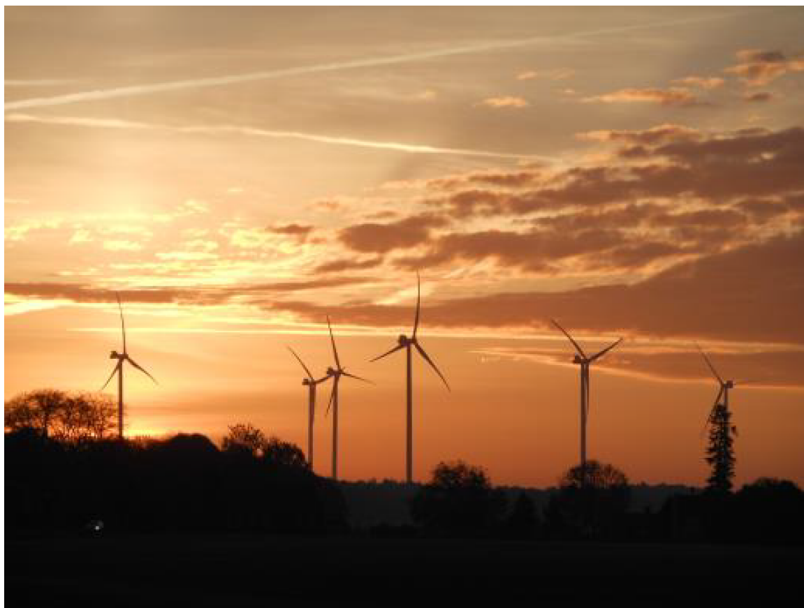
Aftenbillede fra Windpark Rossau (33 MW). Idriftsat medio 2013-primo 2014. Evening shot from Windpark Rossau (33 MW). Operations started mid 2013-beginning 2014.
