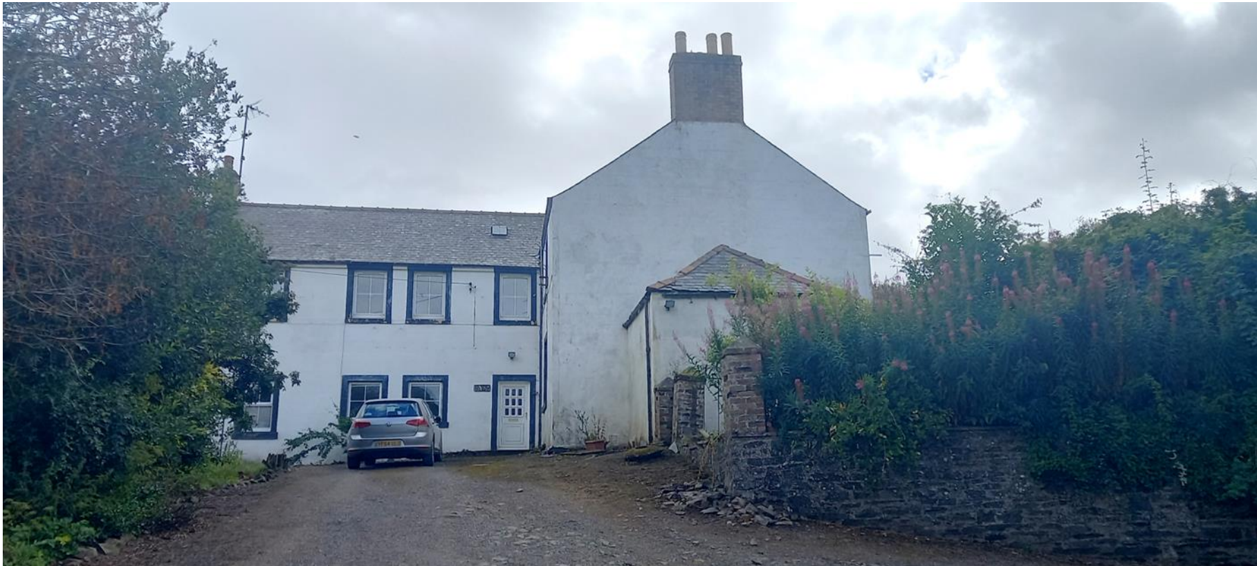
Plate 19: Front elevation of Howpark Farm House (LB46642)
